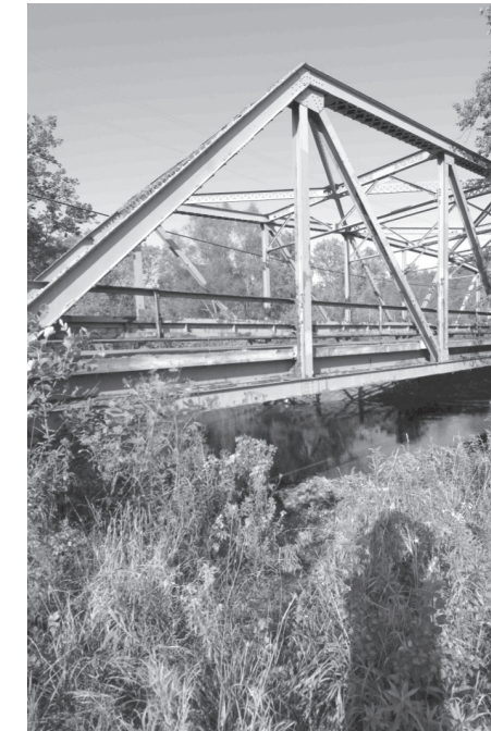
Compton Bridge on County Highway 11C Photo credit: R. Walker
